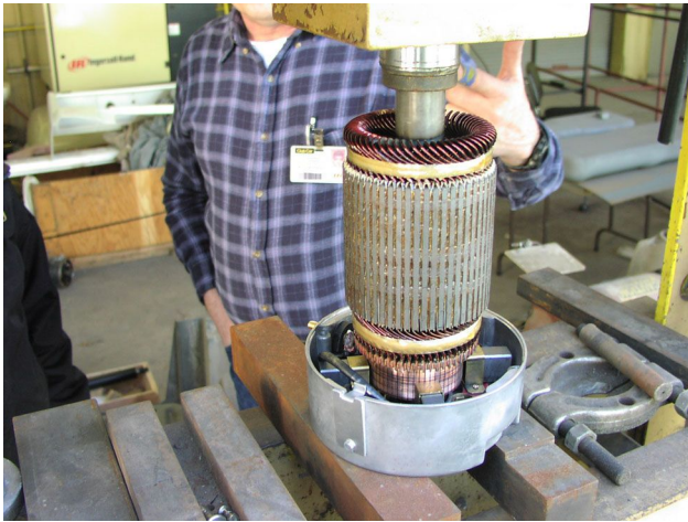
Figure 23-18 Armature Installation
